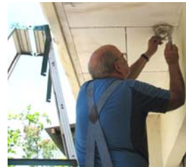
Russell Conrad working on the electrical system
