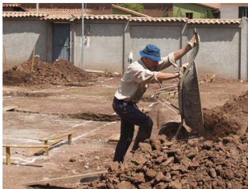
Rob McEwin working on foundations
